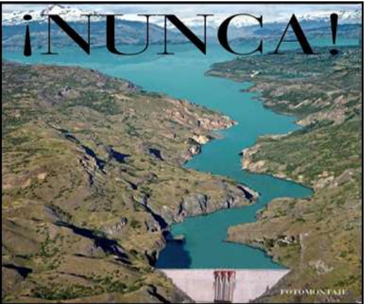
Hydro Aysen 2.3 GW Dam Project
